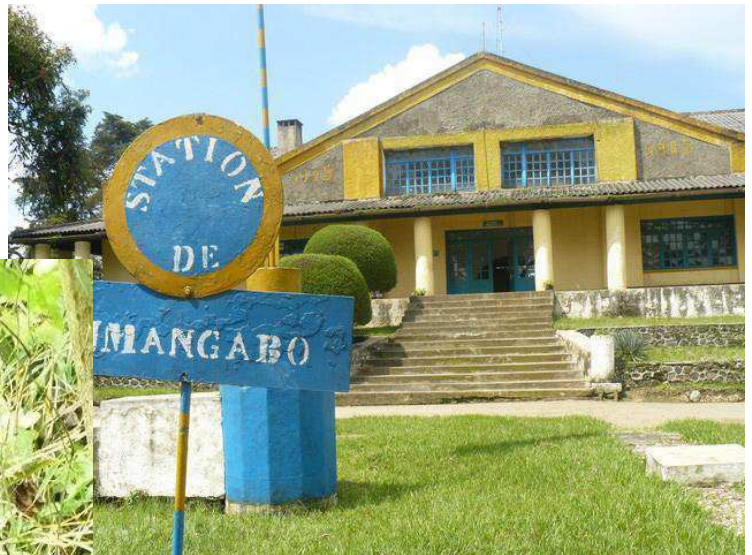
The main administrative building of the Park
